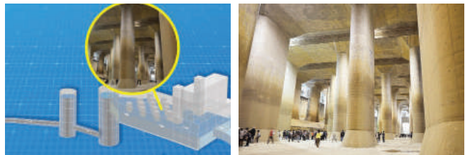
Tokyo's Underground Tunnel
