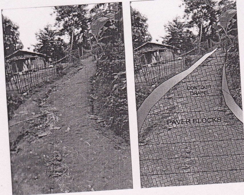
Figure 6.3 : Illustration of a contour drain at site
