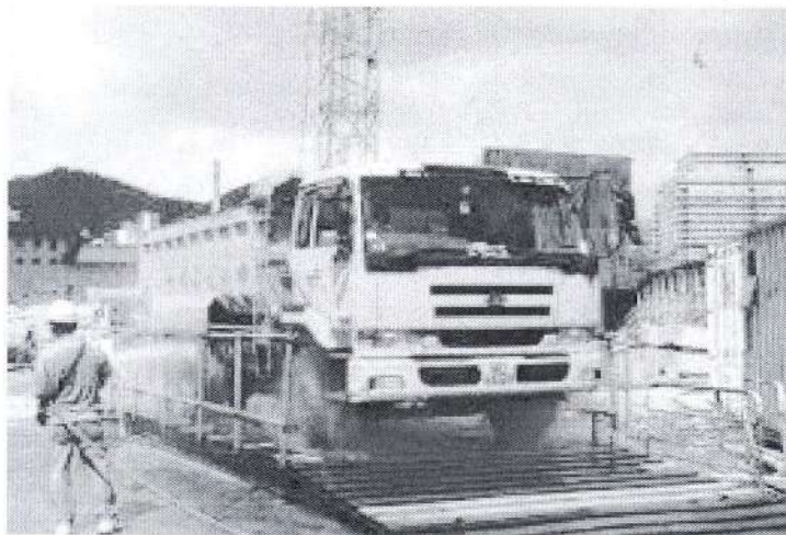
Figure 6: Washing the wheels of vehicles with dust suppressants
