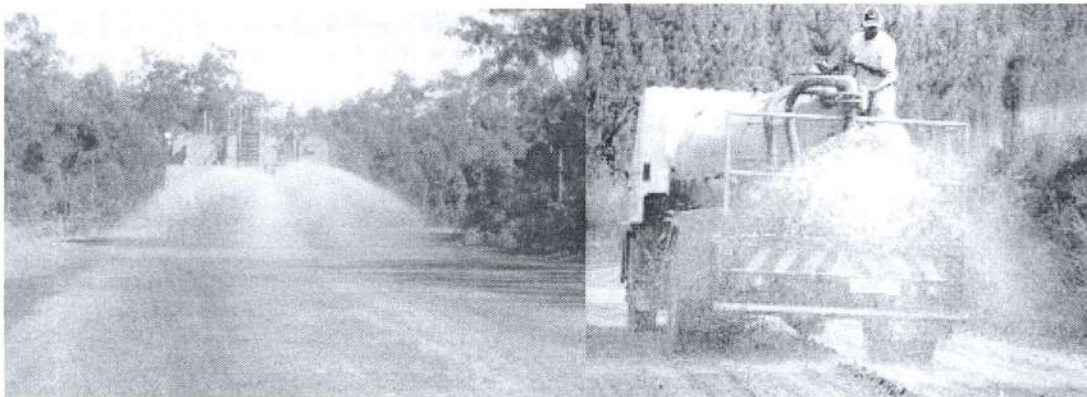
Figure 4: Application of dust suppressants for unpaved roads
