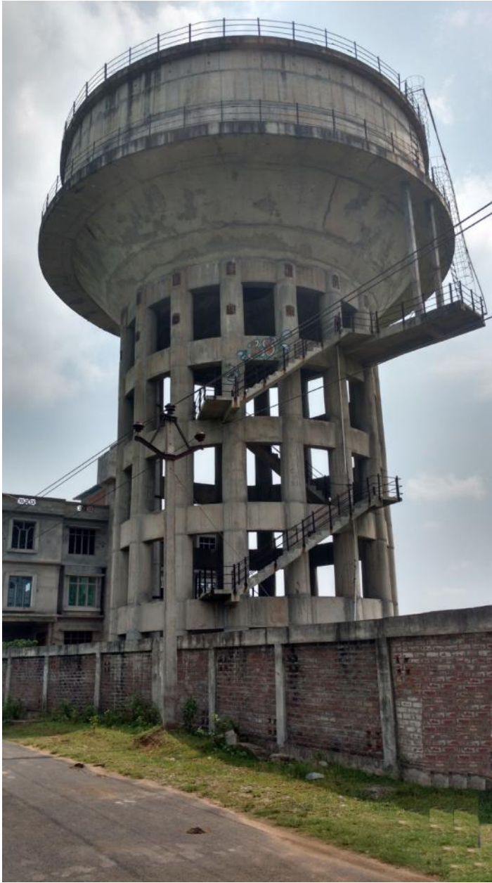
ELEVATED SERVICE RESERVOIR OF CAPACITY 16 LACS LITRES EACH AT BORJHAR & MIRZAPUR.
