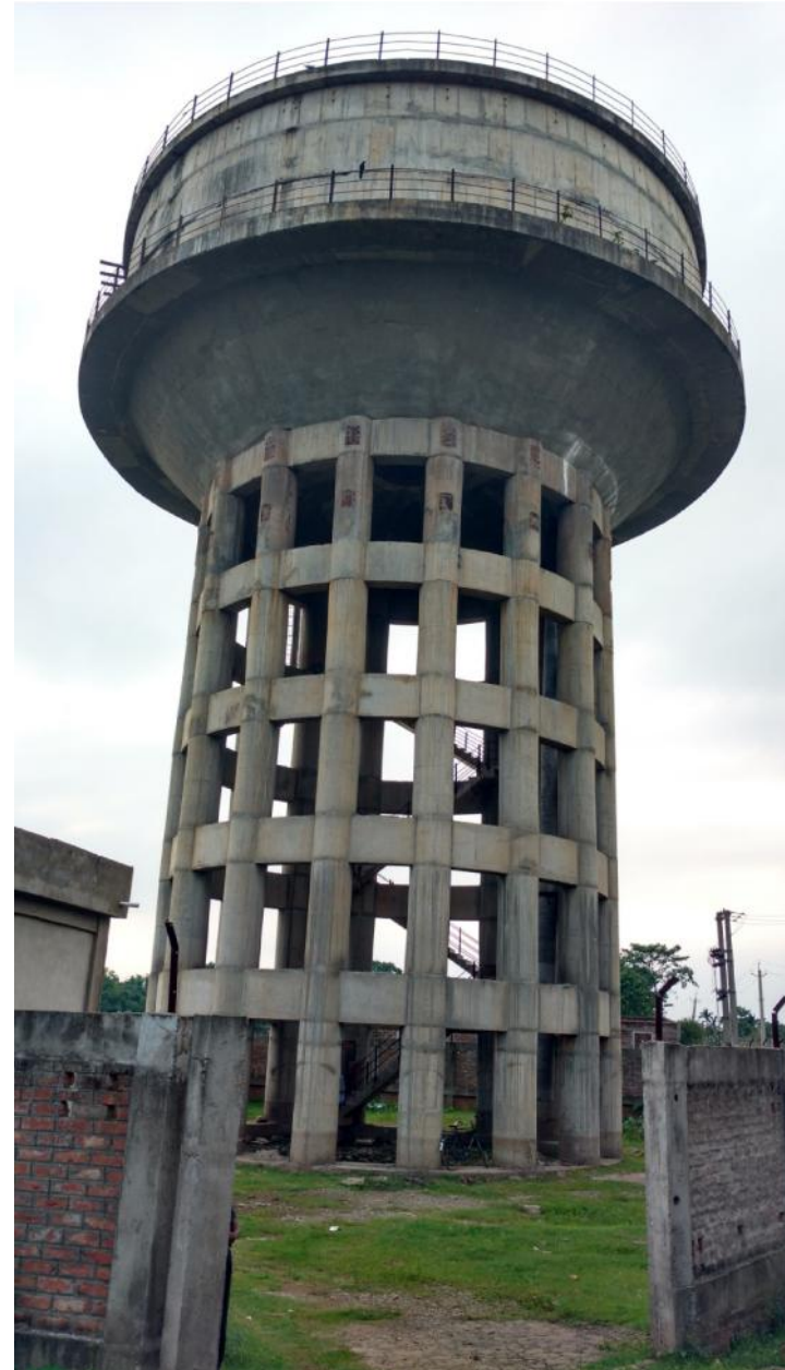
ELEVATED SERVICE RESERVOIR OF CAPACITY 16 LACS LITRES EACH AT BORJHAR & MIRZAPUR.
