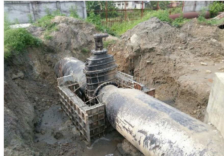
SAMPLE PIPE LAYING / VALVE INSTALLATION
